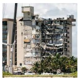
oceanfront beach property always exposed to salt-spray. Salt causes corrosion in reinforced concrete structures. This in turn causes structural deterioration. Failure in repairing this deterioration eventually compromised the building structure which then collapsed.
