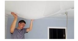
You purchase a clothes washer or dishwasher that gets installed incorrectly. A tube pops off and water leaks through the floor to the unit below. No water sensor systems were installed. There is no visible evidence of a leak until the frantic owner below calls management about water leaking through their ceiling.
