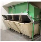
Your building's waste disposal system has heavy demands. On a daily basis residents dump their trash, recycling and organics waste down metal chutes that end in the trash room. Chutes get coated with waste from unbagged or
