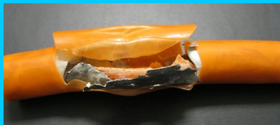
Pipe Damage from Kitec Blowout
